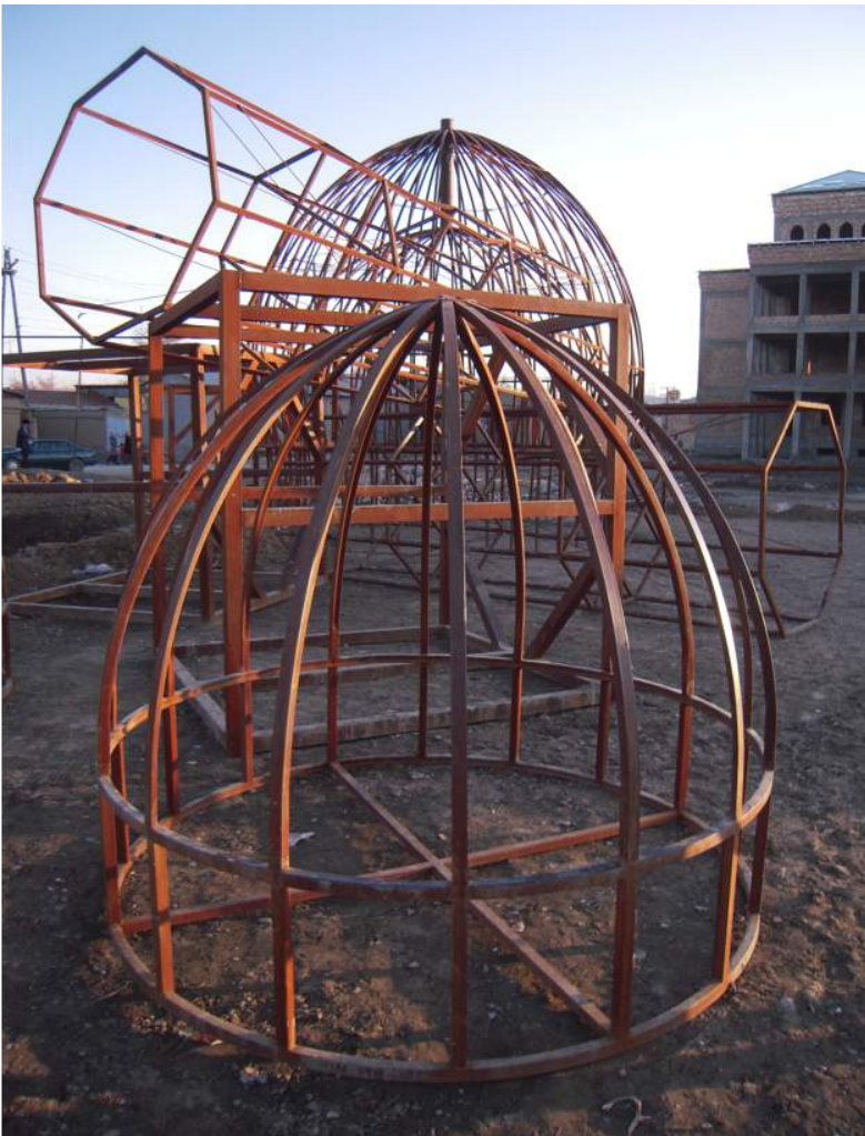
Dome frames near an unfinished madrasa
