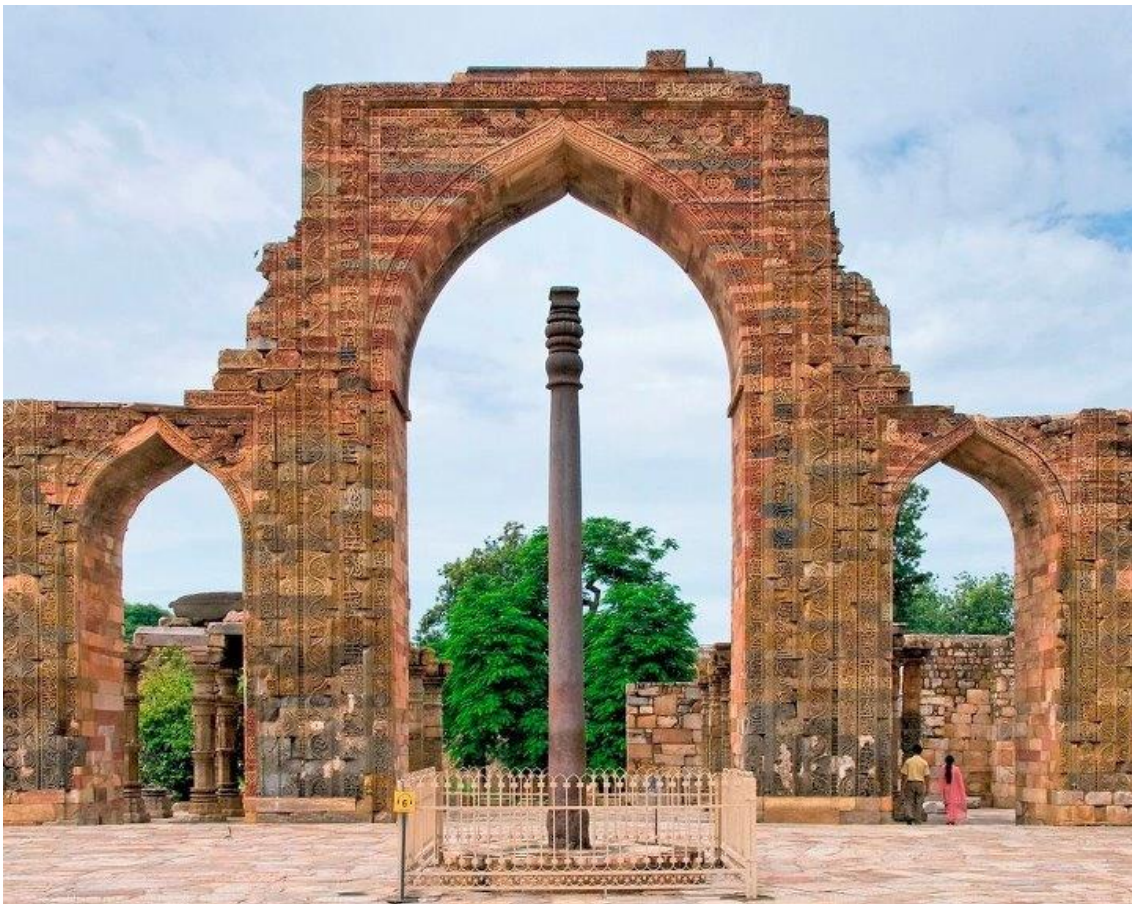
Iron Pillar, 3 B.C. New Delhi, India © Prachodayat
