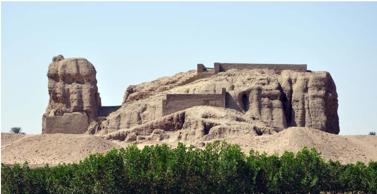
Figure 1 | The western deffufa with the new wall built at its top.
