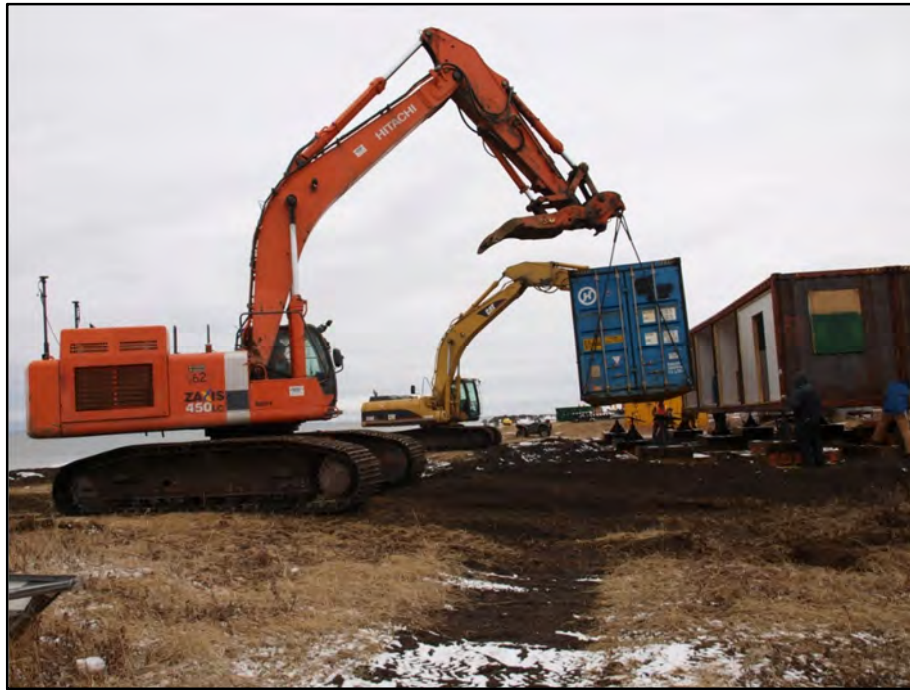
Figure 3: The construction of the new health clinic in Kivalina 2009.
