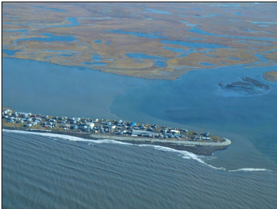
Figure 2. Aerial view of Kivalina August 2009. The new rock revetment or seawall is visible on the foreground. It was designed to protect the village from high waves and erosion.
