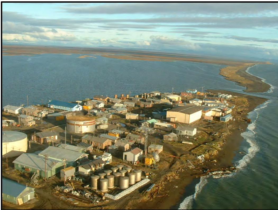
2008: Erosion has been severe on the ocean side. Courtesy Millie Hawley, Kivalina.
