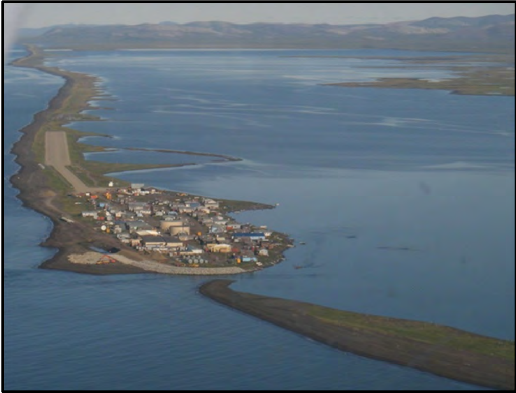
2009: The first portion of the erosion protection is finished. The construction has been halted due to lack of funding. Courtesy Millie Hawley, Kivalina
