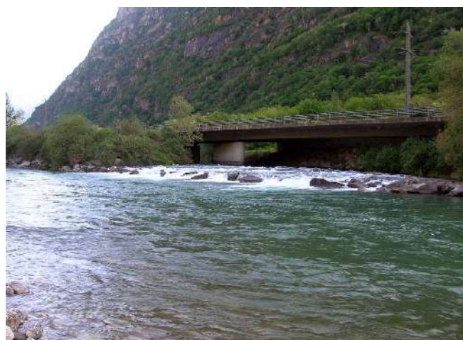
Fig. 2.35. View of the channel releasing water used for hydroelectricity in Lodrino.
