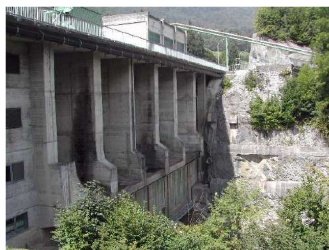
Fig. 2.15. View of the Lessoc dam.
