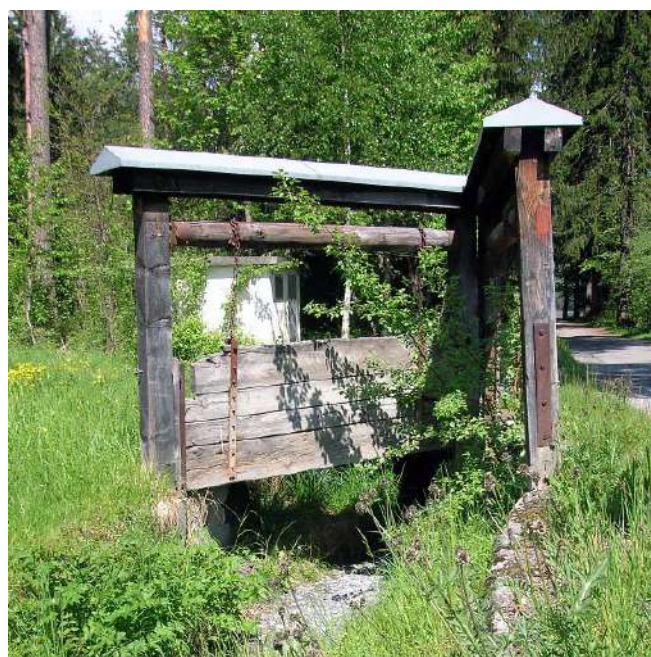
Fig. 2.31. Views of “Nollakanal” still using nowadays by the Realta exploitation.
