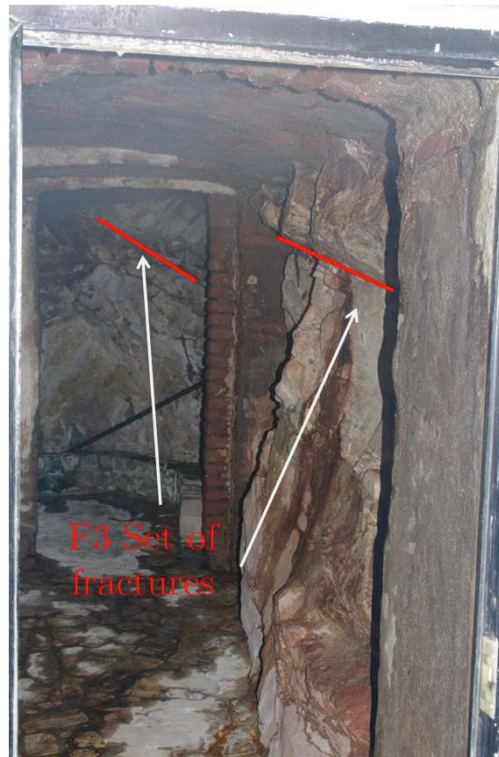
Figure 4-11 Detail of one of the thermal springs' cave where the low angle F3 set of fractures cuts the fine grained granite in correspondence of the thermal springs
