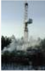
Geothermal research lab, Gross-Schönebeck, Germany
