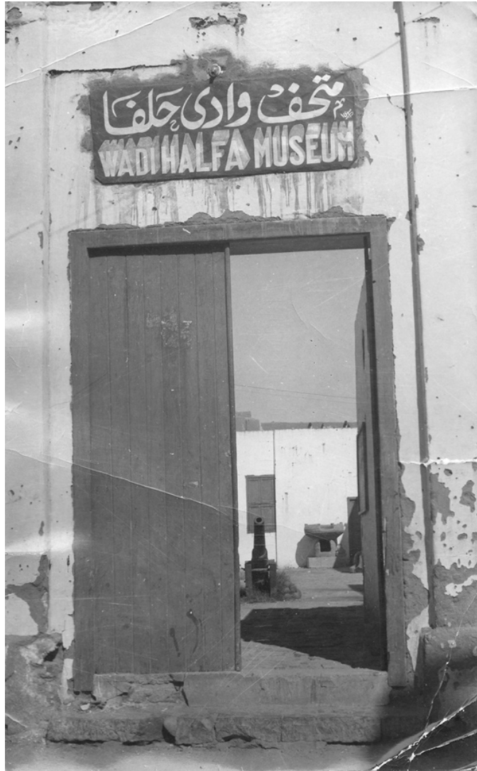
Wadi Halfa Museum, at the premises of the former Merkaz Buildings.
