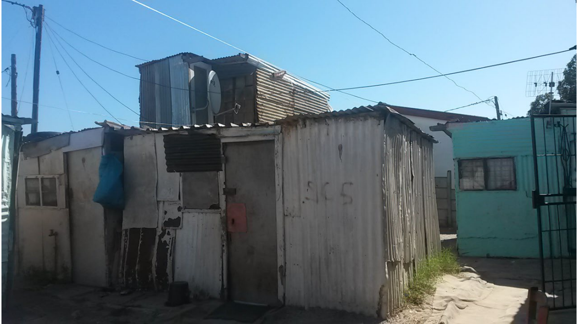
FIGURE 23 SC structures with improvised water tap connection [JB]
