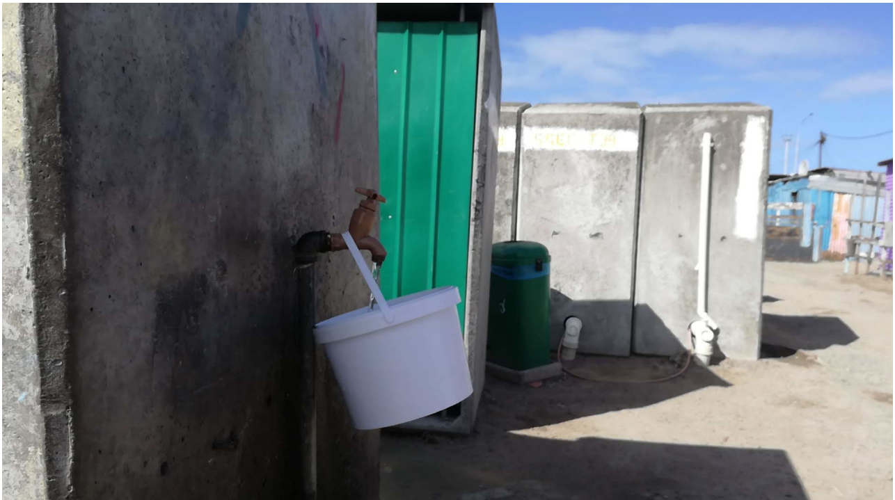
FIGURE 22 CoCT taps and toilets in the SC sub-section [Altamore S, 2019]
