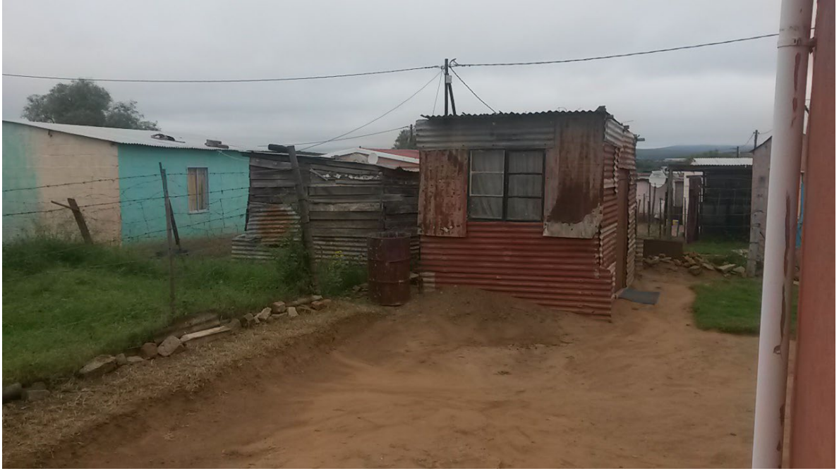
FIGURE 60 Backyard shack in BNG housing near Fort Beaufort (Eastern Cape) [JB, 2018]
