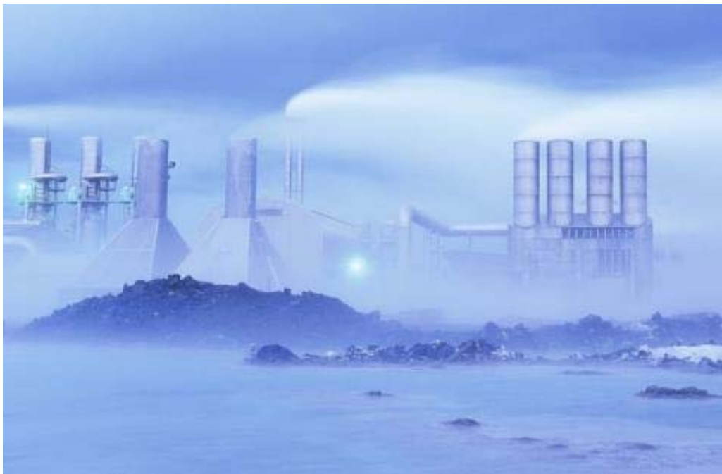
Photo 1: The Svartsengi geothermal power plant by the Blue Lagoon in Iceland. (Photograph: Paul A. Souders, Corbis)
