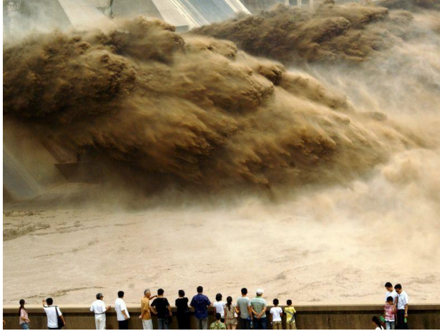
Figure 17. Sediment Flushing of Reservoir Xiao Langdi, China (Photo source: The China Times).
