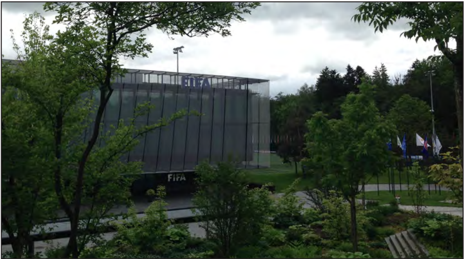
Figure 6: Fédération Internationale de Football Association (FIFA) headquarters in Zurich, Switzerland.
