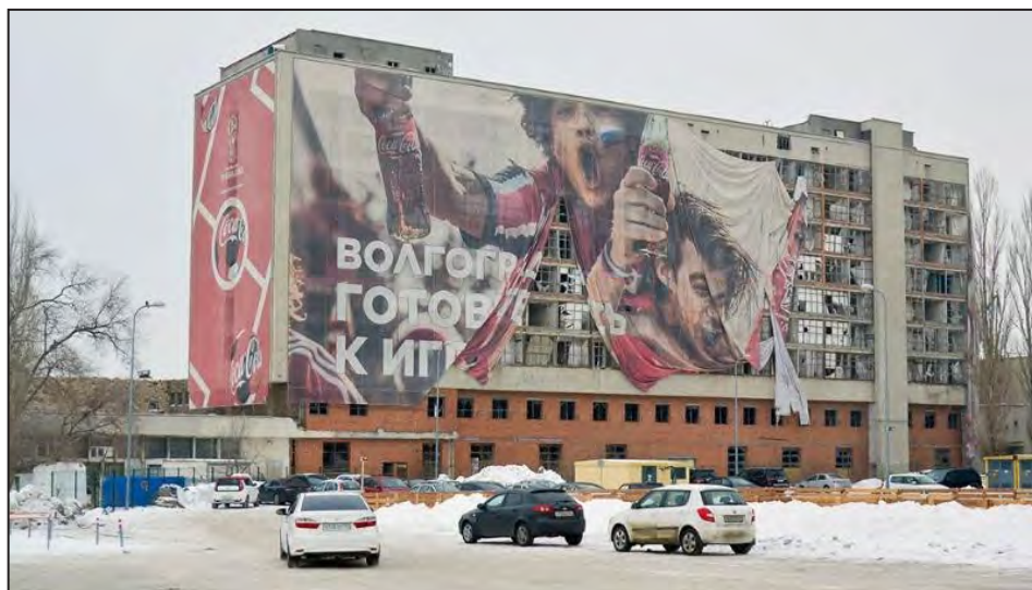
Figure 38: Potemkinism uncovered: abandoned building in Volgograd with a Coca-Cola building wrap that read “Volgograd! Get ready for the games!” Source: Viktor Yastrebov
