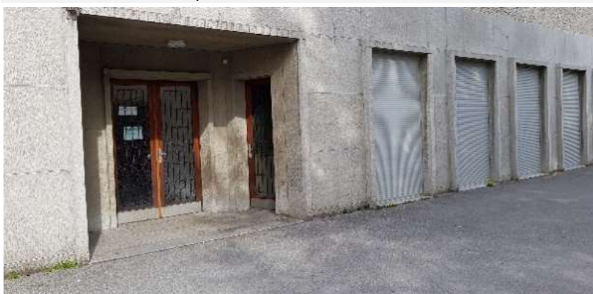
FIGURE p Entrée grande salle
