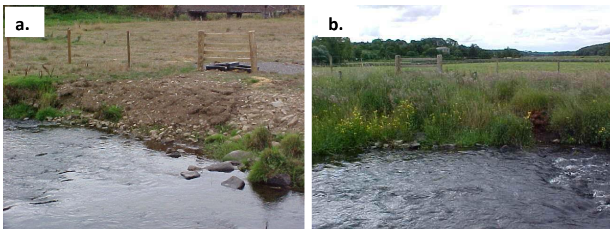
Figure 4 Fencing and bank restoration at Chapelhaugh near Methlick in the Ythan catchment. The banks had been heavily eroded pre-restoration. a. Fencing and bank restoration done using felled conifer logs b. regrowth of native vegetation and stabilized banks Source: Ythan project, retrieved from ythan.org.uk on August 4, 2014.
