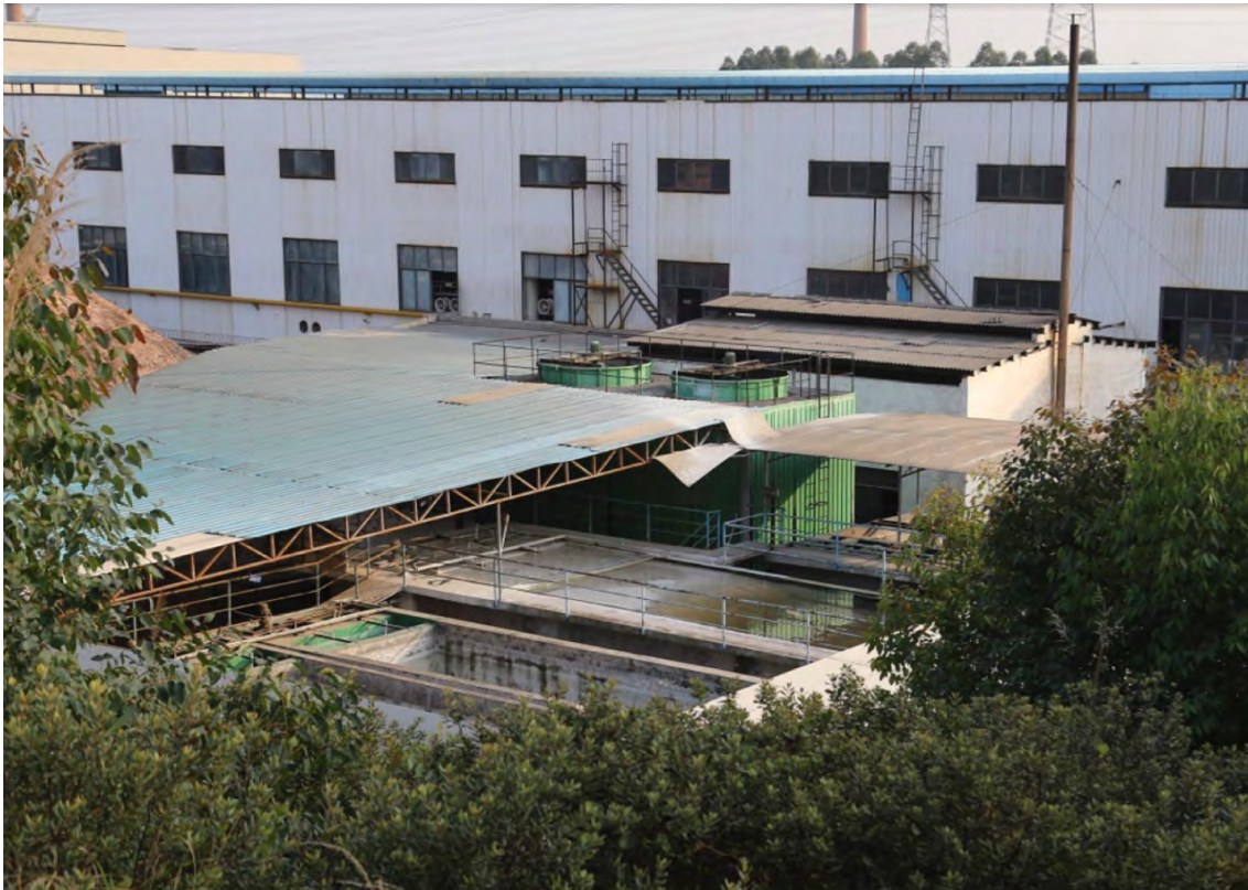
Figure 4.14: The water treatment facility in Huaqing's industrial park. Photo credit: the author.
