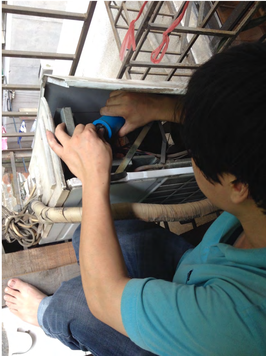
Figure 7.2: This repairman fixed my air conditioner by replacing a component. He sometimes has to climb on building facades to access that type of appliance. Photo credit: the author.
