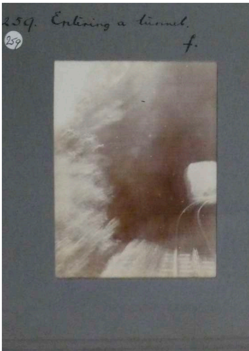
Fig. 10.6 A.H. Fisher, Entering a tunnel . Tratta per Coonoor, Burma, (1907).
