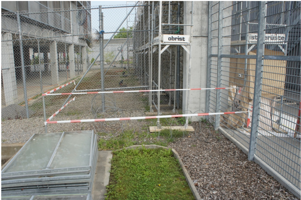
Figure 14: Scaffolds installed on the prison grounds
