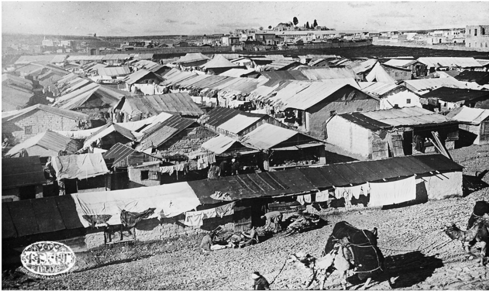
An image from the Aleppo refugee camp in the 1920s shows makeshift houses made of mud bricks, tin cans, wooden crates, and canvas. The "housing famine" made obtaining housing a major issue that Jeppe sought to solve with the construction of a new compound in Maydan outside the city center (Source: The Karen Jeppe Archives, Gylling, Denmark. Courtesy of Mihran Minassian).
