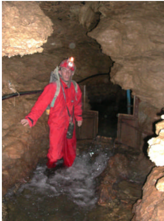
Figure 23: the Milandrine upstream weir at low water stage. The dark pipe behind is the SO impoundment.
