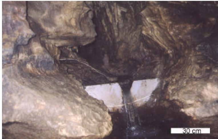
Figure 24: Plastic weir constructed at RO tributary in order to measure continuously discharge with a water level probe.
