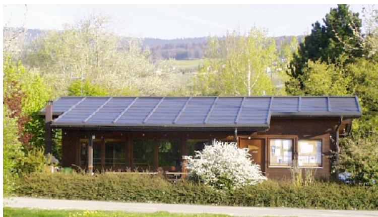
Fig. 1.1: Solar roof made of amorphous silicon PV modules, sailing club, Auvernier (CH).
