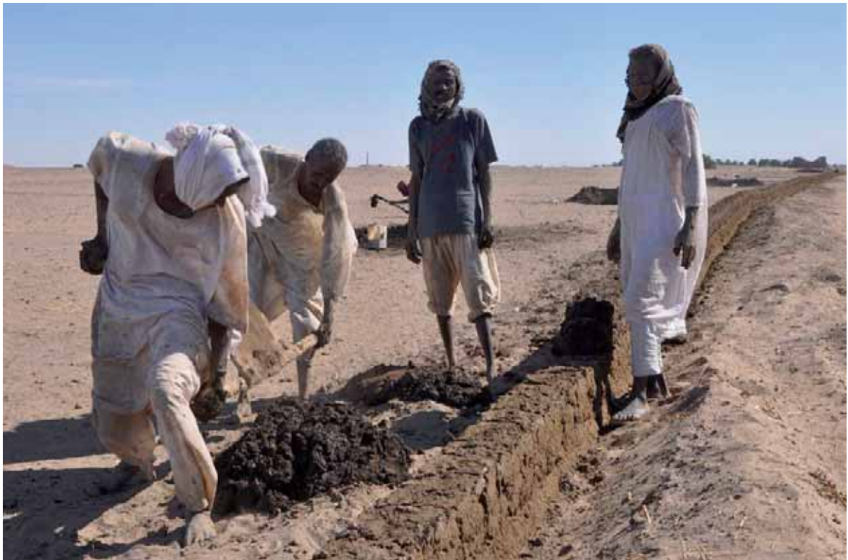
Figure 12 and 13 | Eastern cemetery. Building of a low wall in galous of the western limit of the cemetery in order to protect it.
