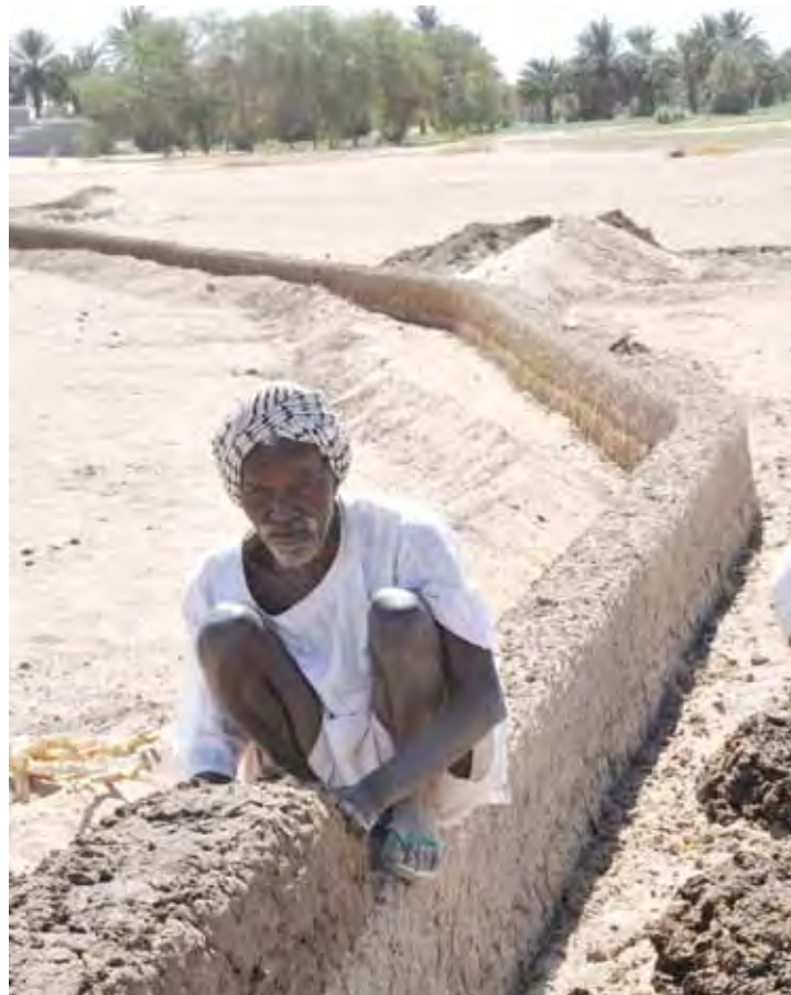
Figure 27 | Protective wall made of galus during construction.
