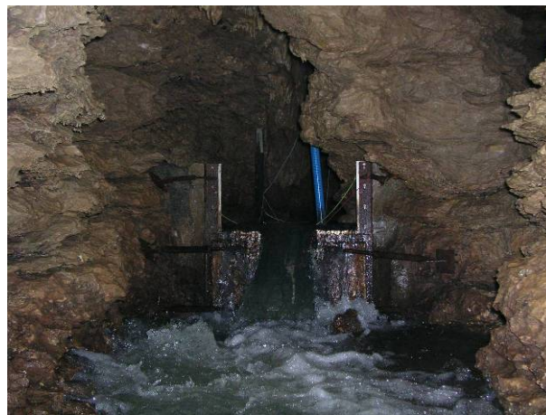
Figure 1.7: Picture of the measurement station in the Milandrine river.
