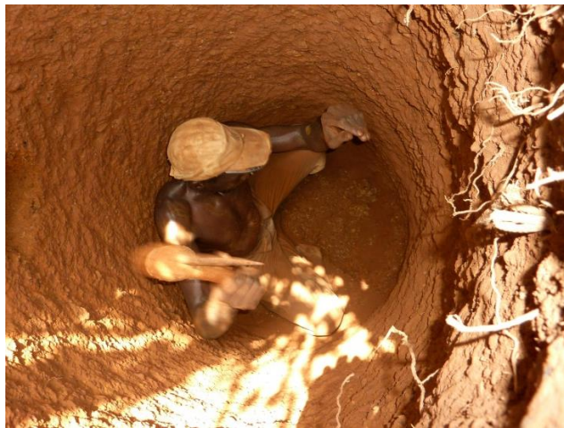
Picture 1-2 Excavation of the vertical well to the deposits (Kintinian, Guinea)
