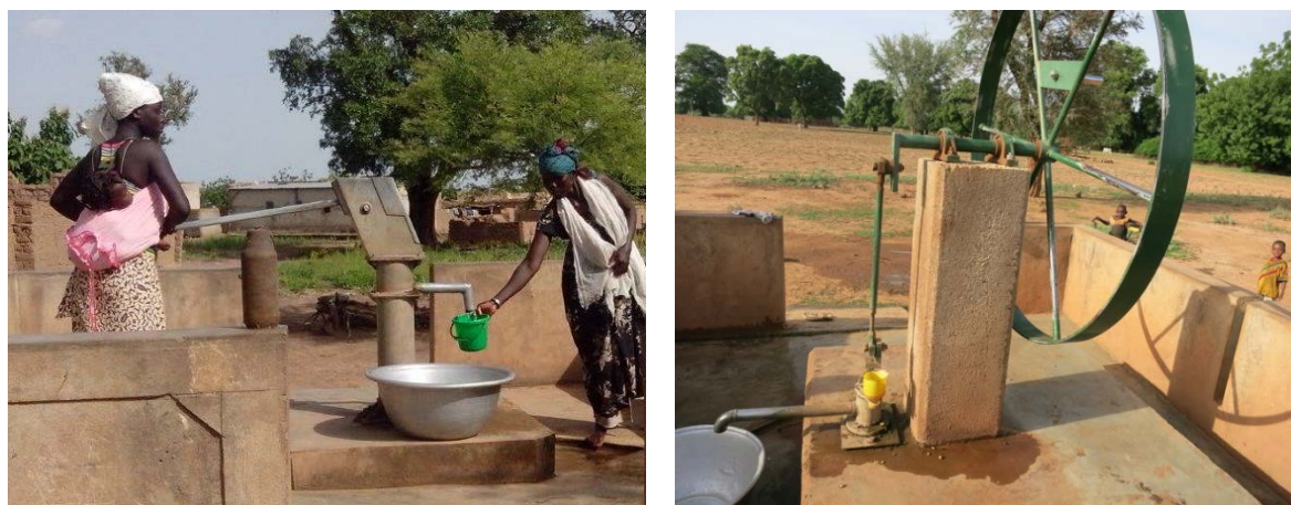
Fig. 1.2 Examples of hand pump types commonly installed in tube wells in Burkina Faso. The picture on the left shows an “India” hand pump, on the right a “Volanta” hand pump.
