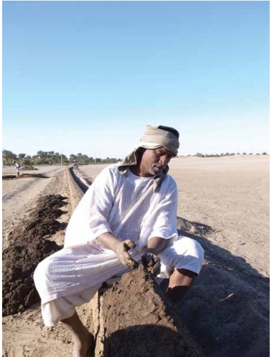
Figure 39 / Construction of the enclosing wall by Awadalla Khalifa Osman and his team. Kerma, royal cemetery.
